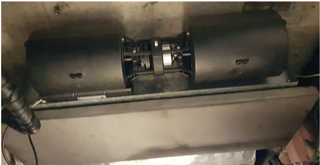
Figure 4.45 Conventional FCU fan and motor replaced with an integrated EC motor
