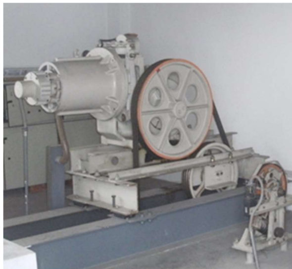
Figure 7.6 Arrangement of a geared drive
