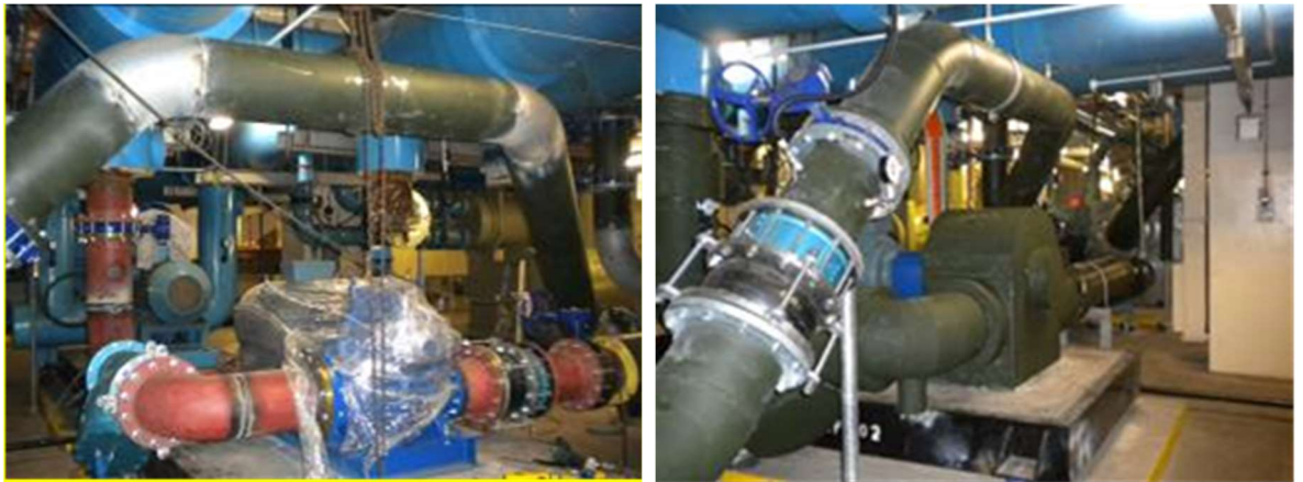
Figure 5.12 Use of long radius bends to reduce pressure losses
