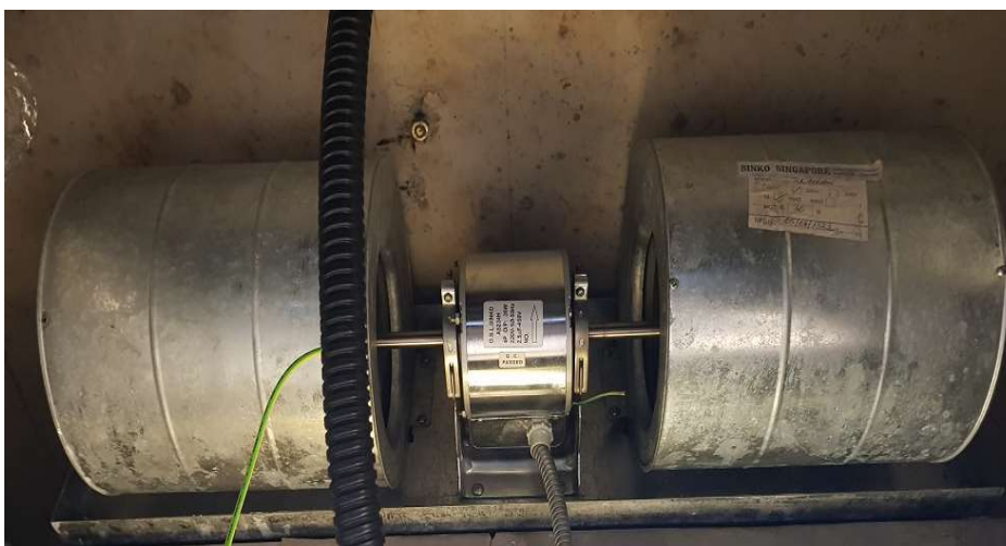
Figure 4.43 Conventional induction motor FCU fan
