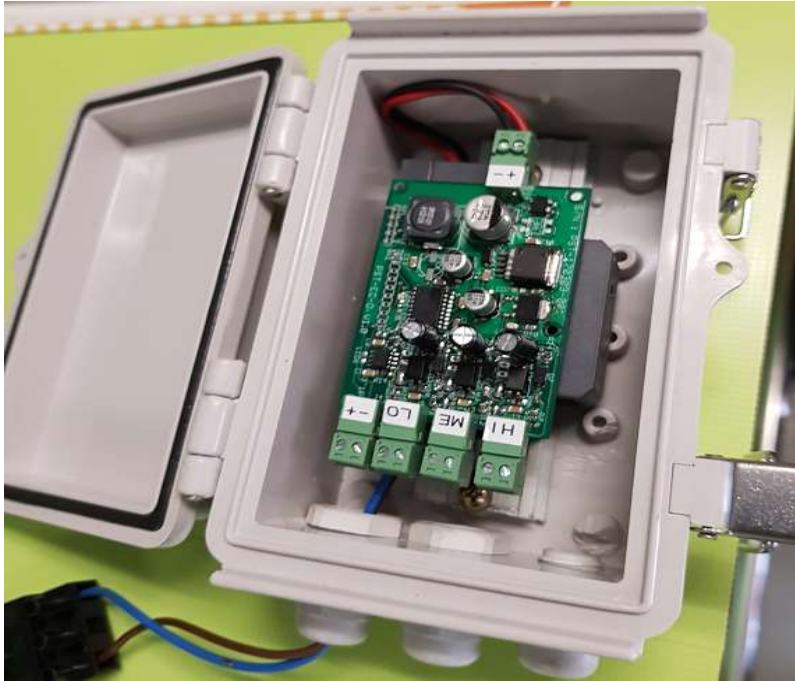
Figure 4.46 Converter box for FCU fan conversion
