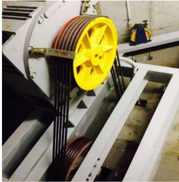
Figure 7.7 Arrangement of a gearless drive
